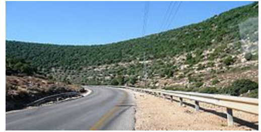
Road in the West Bank
